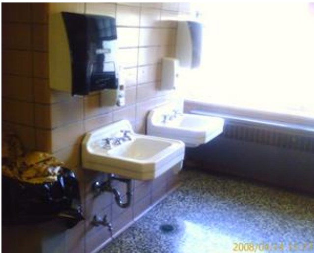
Typical fixture condition
