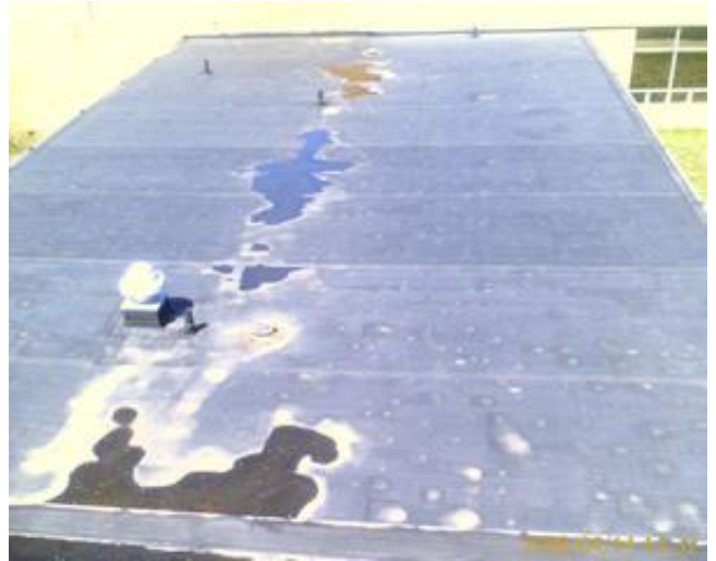
Typical roofing condition
