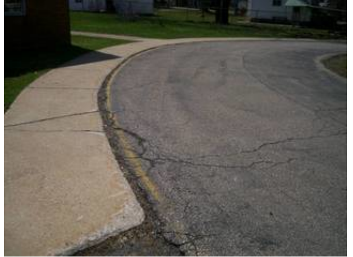
Sidewalk and asphalt pavement
