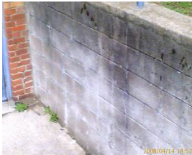
Typical concrete masonry unit foundation wall
