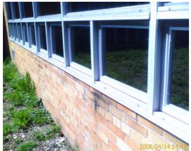
Typical exterior wall condition
