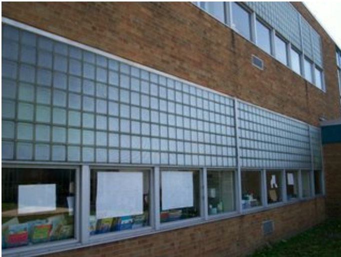
Glass block and single glazed windows
