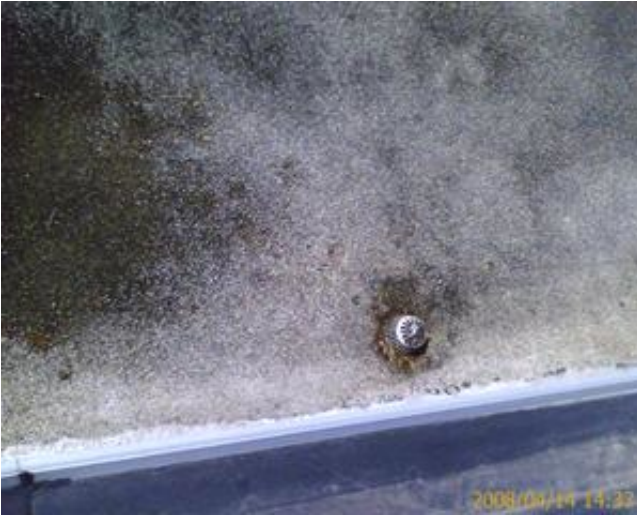
Typical roof drain condition
