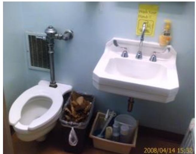
Typical fixture condition
