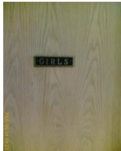
Typical non ADA compliant signage
