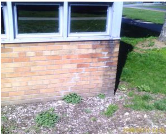
Typical exterior wall condition
